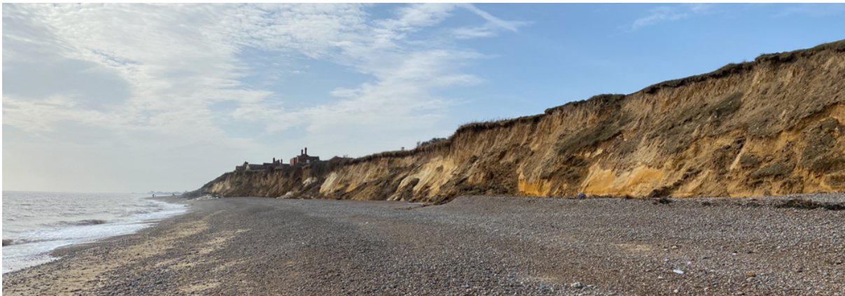
Pillbox 1, just visible on the tideline before the houses on the cliff, is now an estimated 25 meters from the base of the cliff - photo taken in 2021. NB photo taken just south of the site of Pillbox 2.
